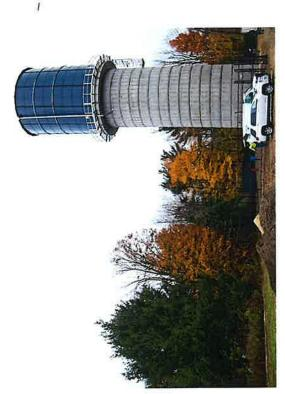
Elevated glass fused steel tank. Paxton, MA 209,000 gallons.
